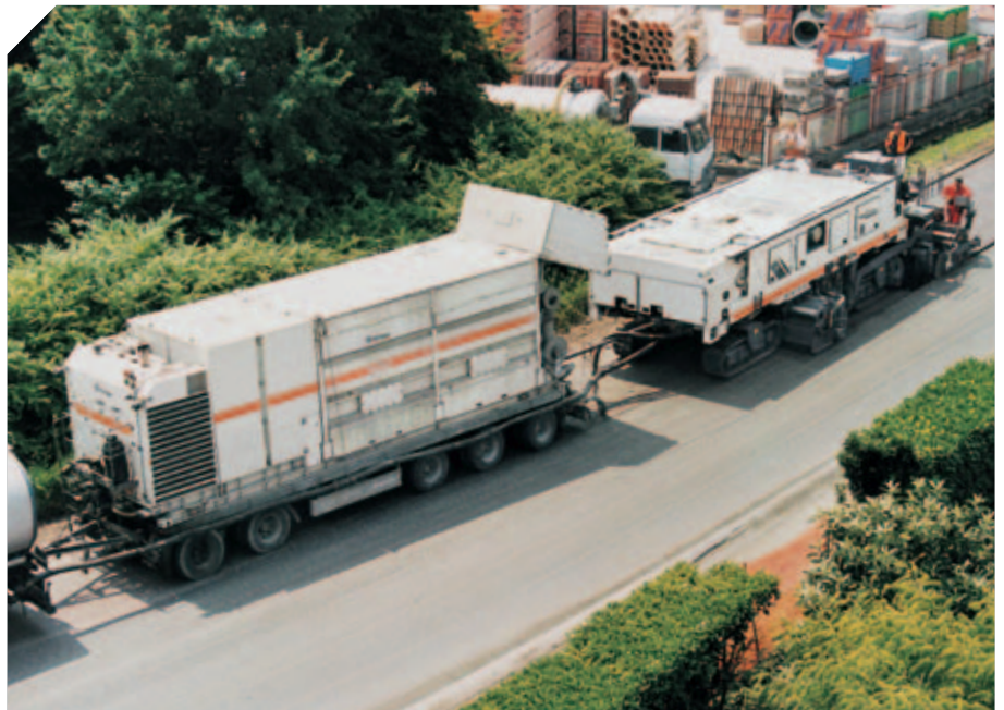
Slurry mixer WM 1000, coupled to the Wirtgen cold recycler WR 4200, rehabilitating a thoroughfare with foamed bitumen and cement.
