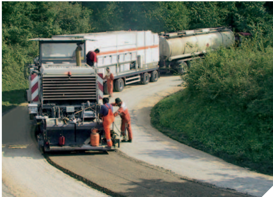
Slurry mixer WM 1000, coupled to the Wirtgen cold recycler 2200 CR, rehabilitating a country road.
